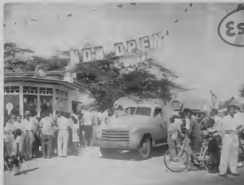
ONE OF the first customers, a soft drink delivery truck, rolls up to a gasoline pump beneath a sign which proclaims the station "Now Open."
